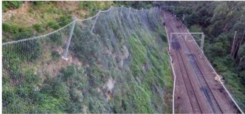
**Figure 2.8:** View of prototype attenuator system installed in Stanwell Park by Geobrugg [13] [GeoBrugg]
