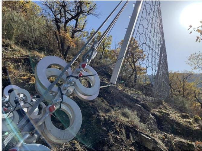
**Figure 2.13:** Detailed representation of dissipation elements [Maccaferri]
