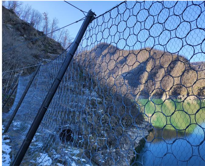
**Figure 2.11:** Detailed representation of interception structure [risp-rockfall protection]
