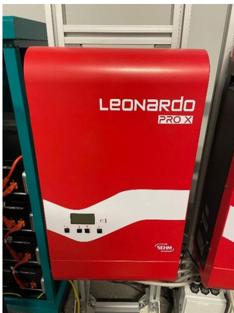
Figura 5-3: inverter Leonardo PRO X 8000/48 Off-Grid
