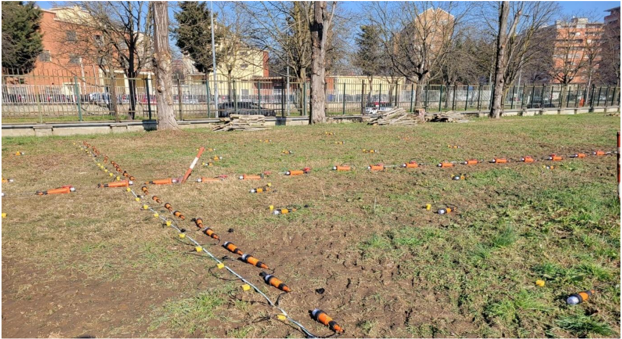
Figure 3-12: Geophysical survey setup at CNR site.
