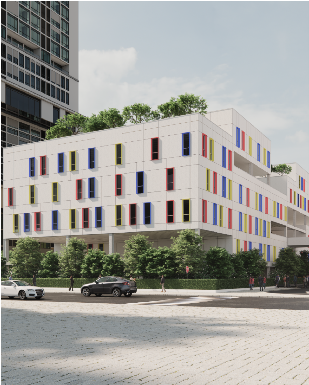
Figure 6.13: Exterior view of the project, Elaborated by authors
