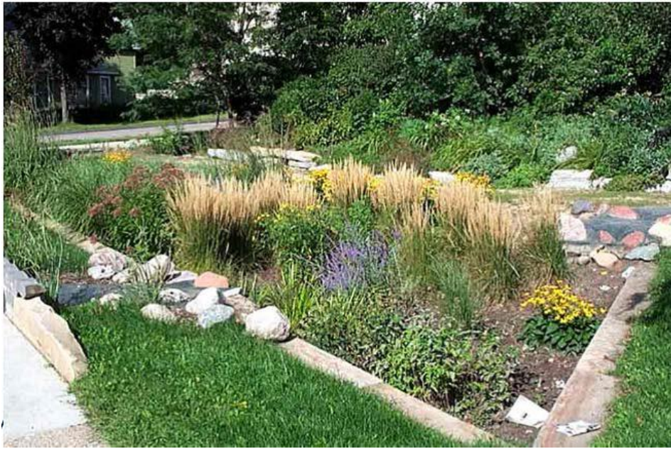
Figure 9: Small-scale rain garden. Source: Andras Kis provided in https://www.nwrn.eu/sites/default/files/nwrn_ressources/u9_-_rain_gardens.pdf
