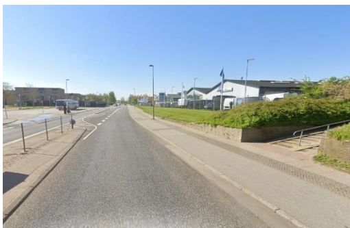
Figure 12, Malmparken Station pavement
