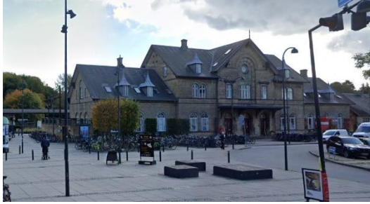
Figure15, Charlottenlund Station surrounding
