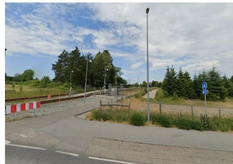
Figure14,Egoje Station surrounding
