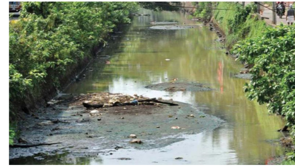
Figure 118 Aftermath of flooding seen in Canoli canal
