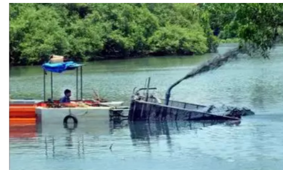
Figure 119 Desilting and dredging works carried out in Canoli canal
