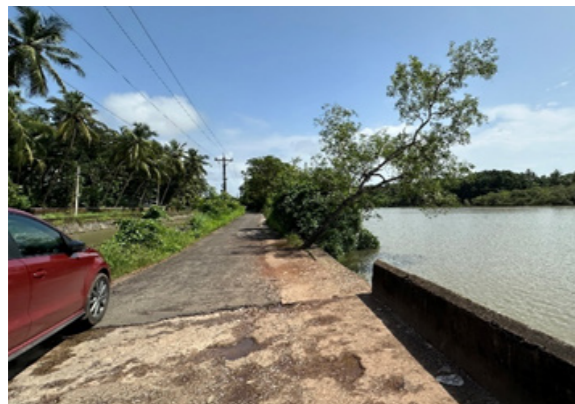
Figure 34 Canal road along Eranjikkal view point (Source: Authors)
