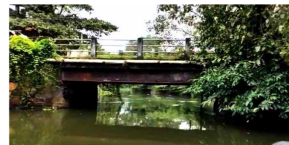
Figure 120 Bridges across Canoli canal with low vertical clearance
