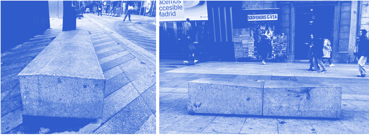
Figure 3. Hostile architecture, example of a bench in Plaza de la Luna with reliefs to limit its comfort.
