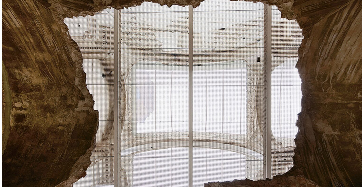
Top: Clear Roof Breathes New Life Into Historic Spanish Church, Corbera d'Ebre in Tarragona, Spain
