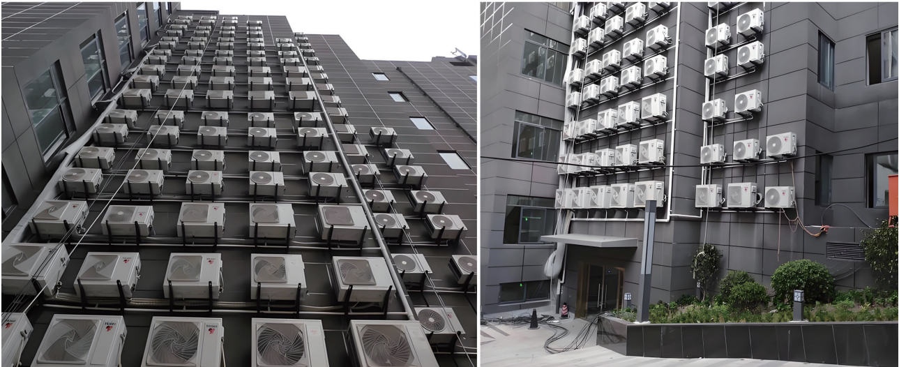
Figure 2.28 The difference between Split Acs and Multi-split Acs
