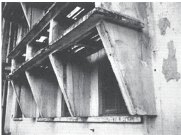
Figure 2.9 Material defects in window shading systems of Xia Changshi
