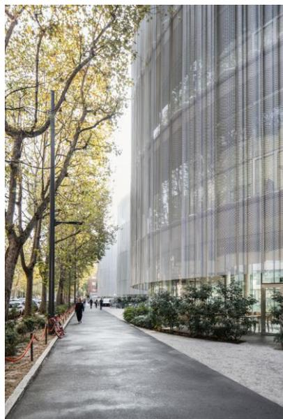
FIG. 2 BOCCONI – SCHERMATURA RETE IN LAMIERA
