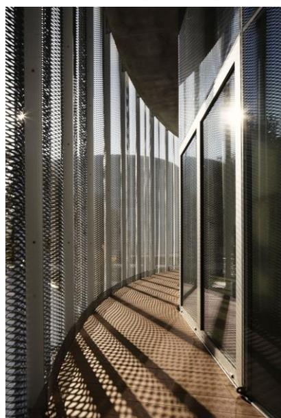
FIG. 3 BOCCONI – SCHERMATURA RETE IN LAMIERA
