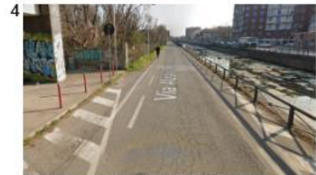
4 Street with discontinuity for active road users.
