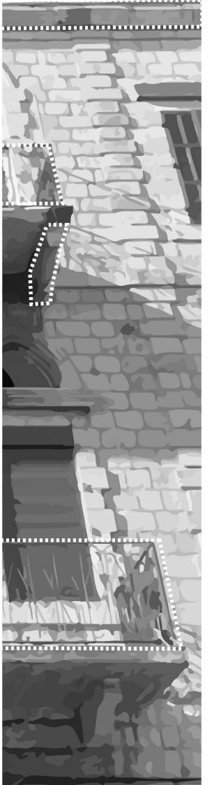
Stone corbels plays an essential part in the Lebanese architectural housings. In terms of functionality, they serve a structural support, anchored into the main structure, holding the balcony. In terms of value, they add decorative importance to the façade providing a visual appealing sight to the observer.
