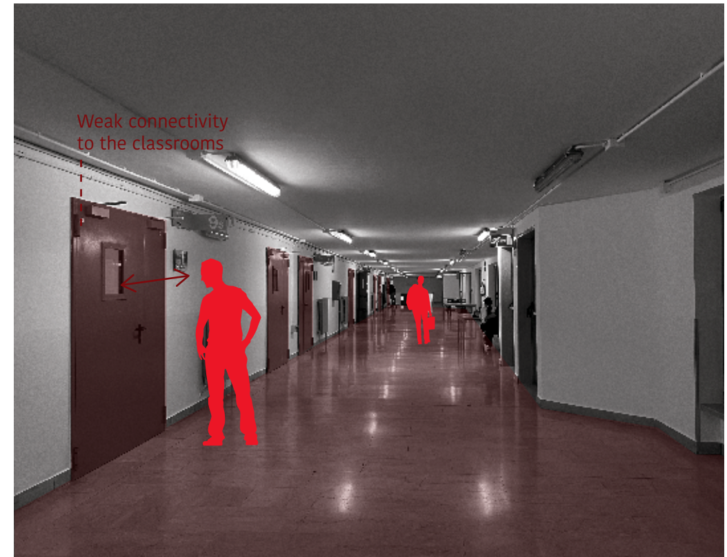
Image 21. Corridor on the basement level on the Main Engineering Campus
