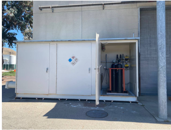
Figure 4.2: Hazardous materials shed containing the N_2O tanks
