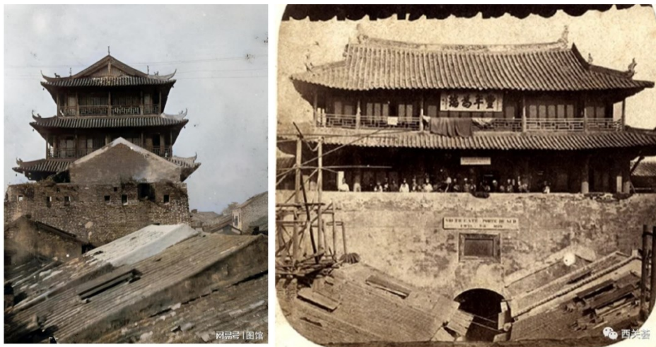
a) DaNan Gate tower
