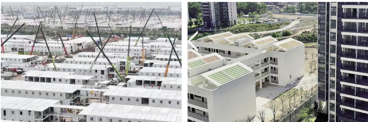
Figure 4-3 Construction of Health Stations in Nansha District
