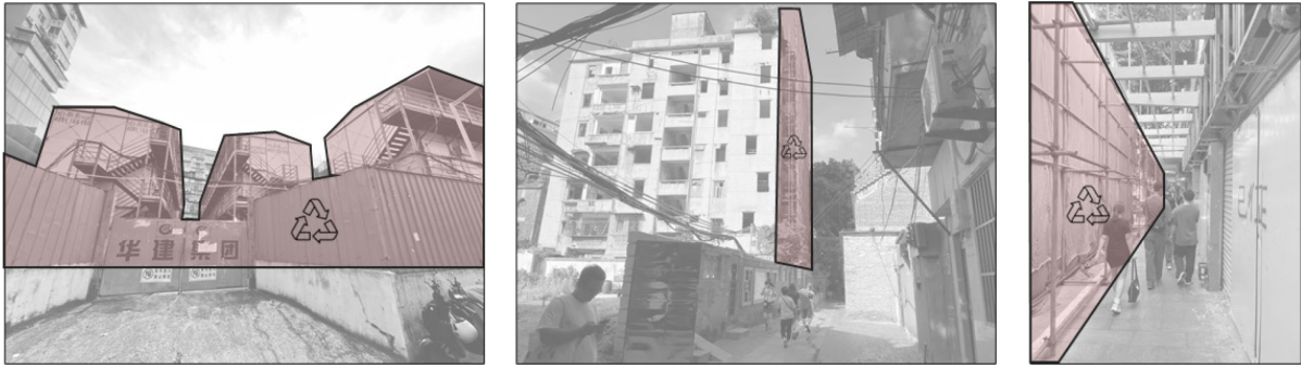
Figure 6-1 Reusable Containers and Scaffolding on the Site
