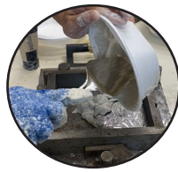
Pouring the mixture of aesthetic outer layer
