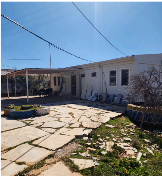
Office section of the facility (Çal 2024)
