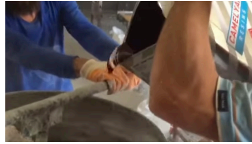
Sixth step, adding resin while the mixing process continues
