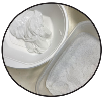
Preparing all materials for the aesthetic outer layer
