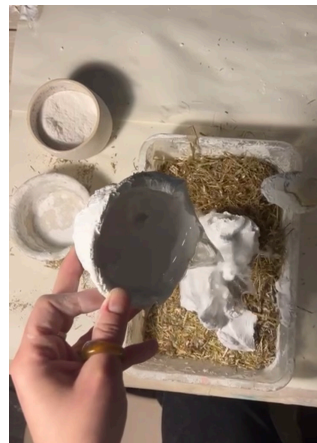
Adding water to hemp hurd and lime putty mix
