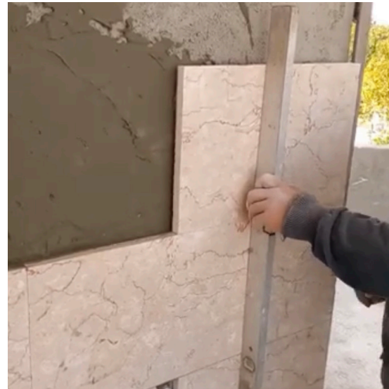
Final step, checking the level
