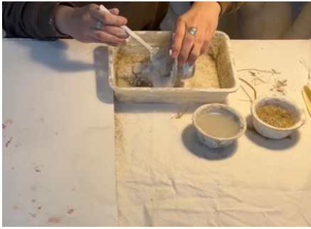
Adding lime putty to marble dust and pouring them together into container
