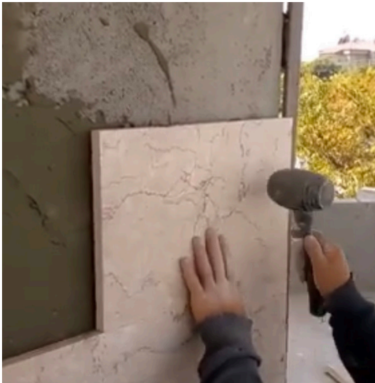
Fifth step, the use soft-head hammer
