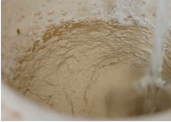
Fourth step, mixing the materials (lime, fine sand, water, pigment, water retainer and fine fiber)
