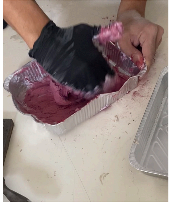
Fourth step, mixing the mixture to obtain Tadelakt as outer layer (Kamis 2024)
