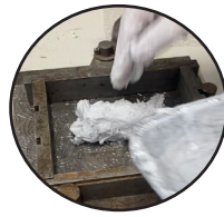
Pouring the mixture of aesthetic outer layer
