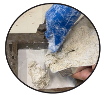
Pouring the mixture of main layer
