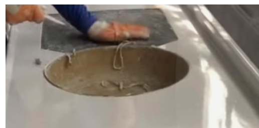
Ninth step, removing the sink
