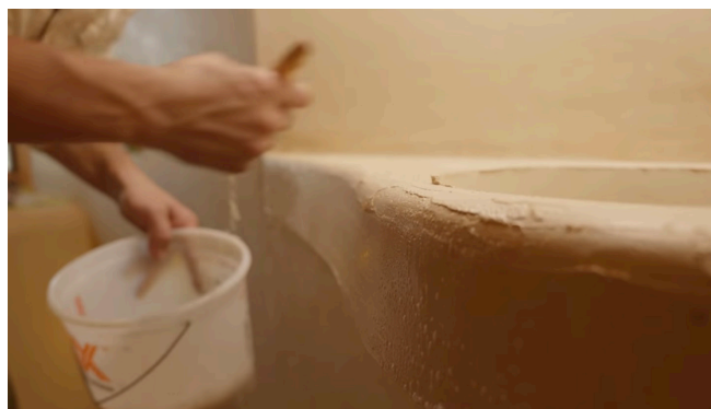
Seventh step, polishing the surfaces with soapy water (20% Moroccan black soap to 80% water)
