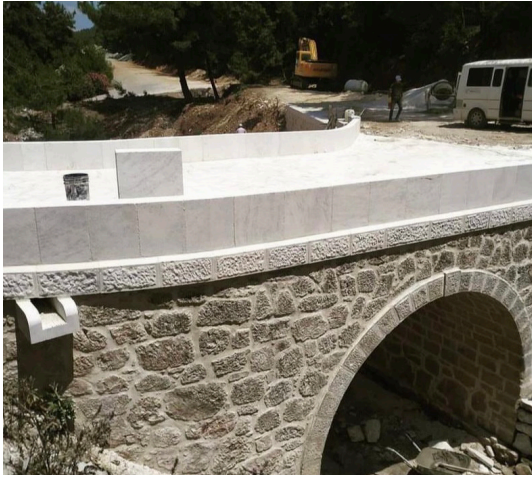
Mugla white marble used in bridge restoration Mugla, Turkey (Bağcı 2019)
