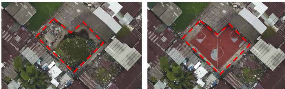
a) Before Renovation
