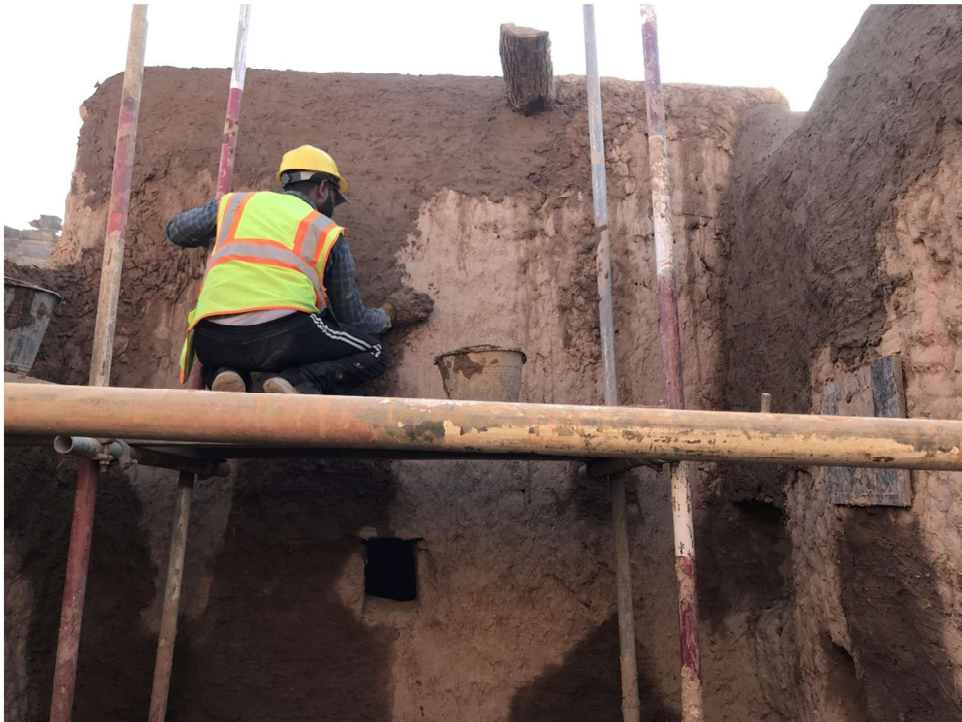
Fig. 07 : Clay implementation on exterior finish face
