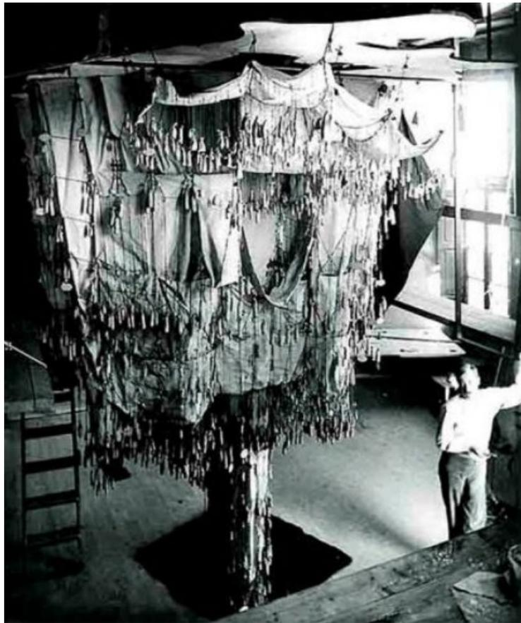
*Fig. 2.3 – Tensile-only model of the Church of Colònia Güell (From: C. Karul (2015), The flexible Fourier form and panel stationary test with gradual shifts).*
