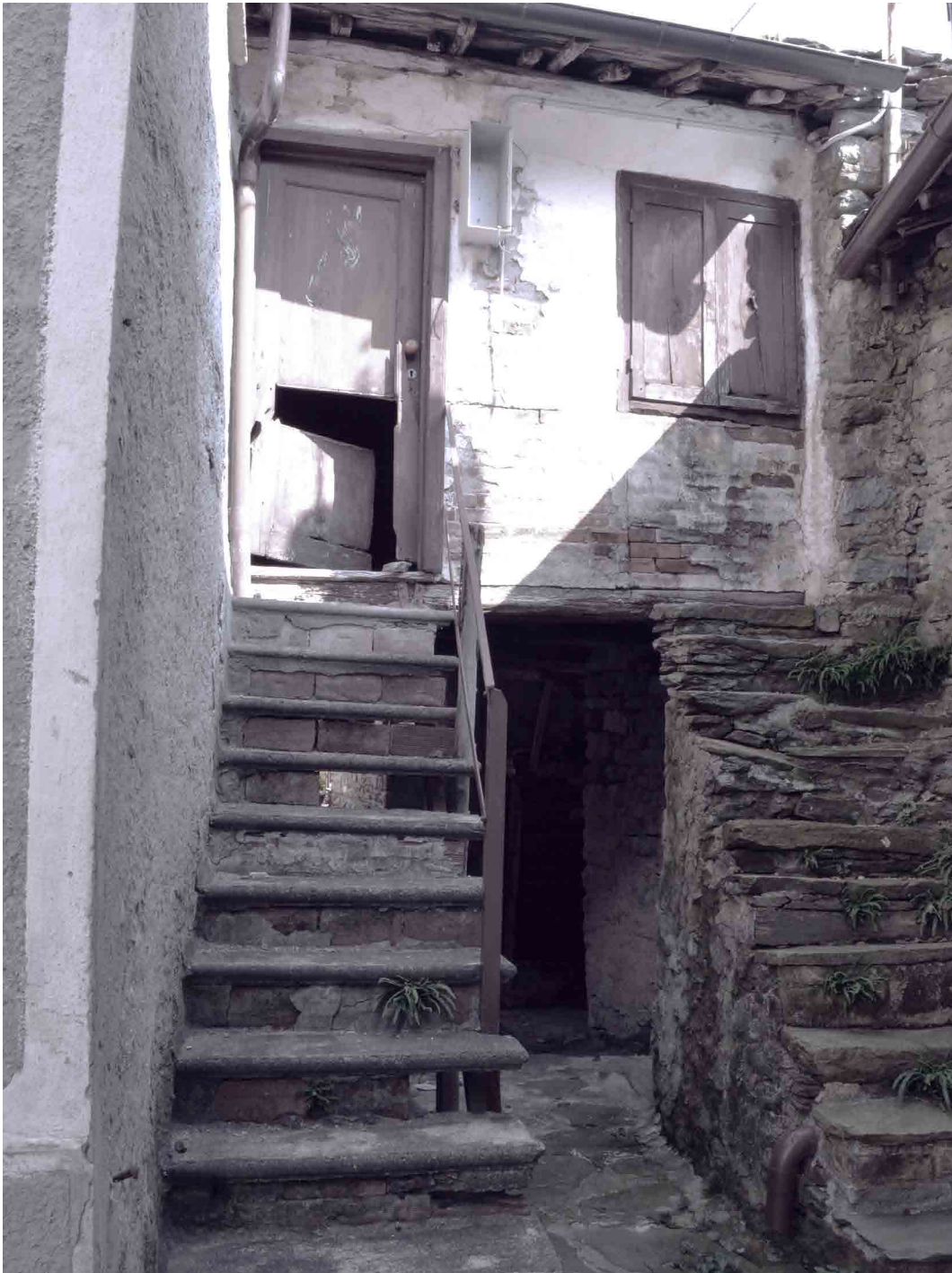
Front South. Photograph taken by the author
