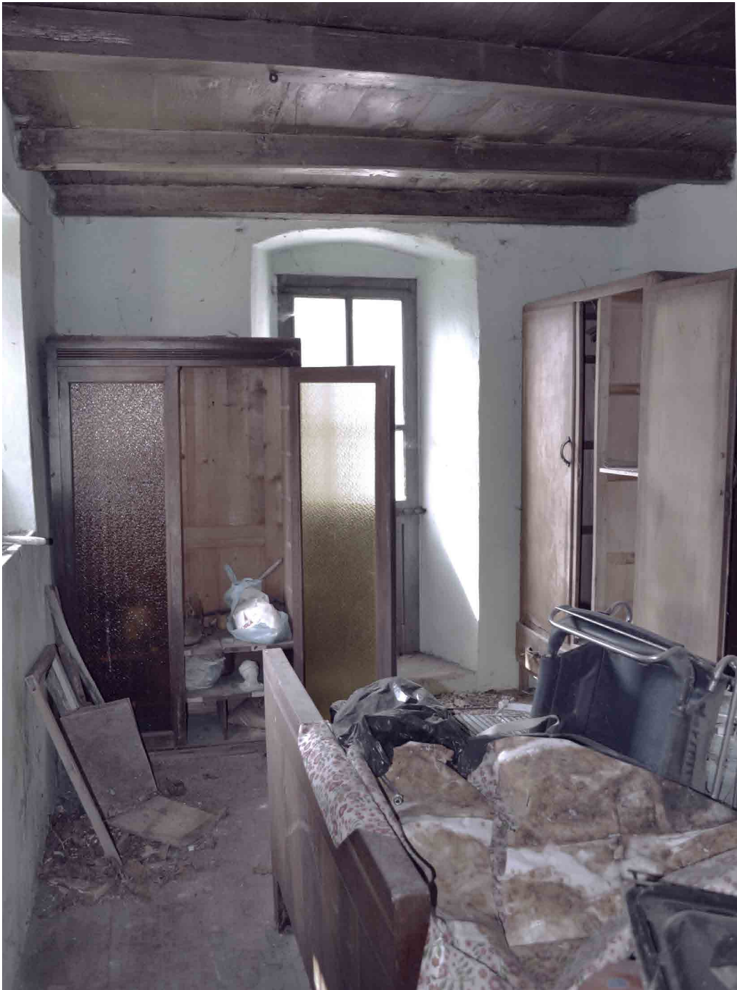
View n°5 First Floor. Photograph taken by the author
