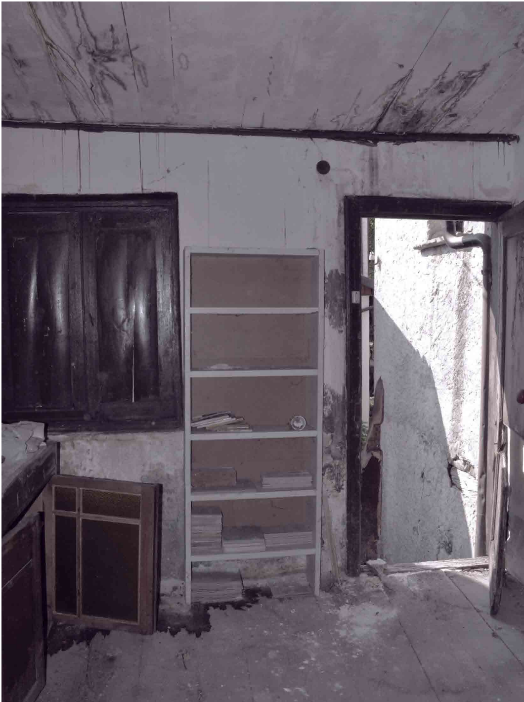
View n°1 First Floor. Photograph taken by the author
