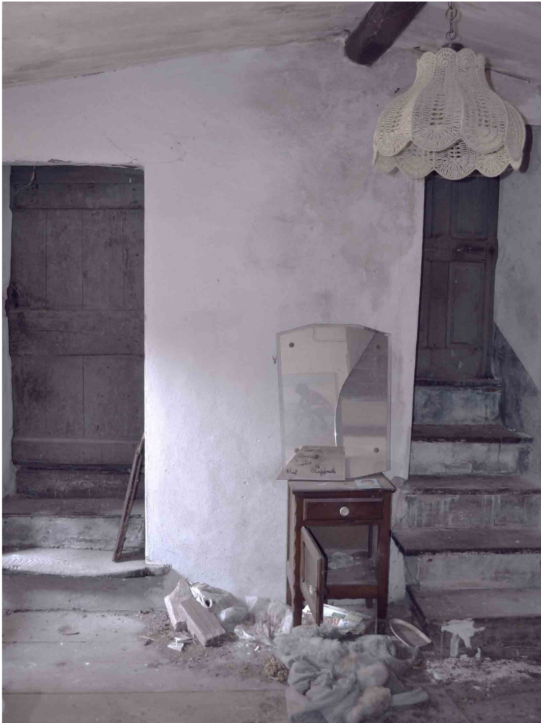
View n°2 First Floor. Photograph taken by the author
