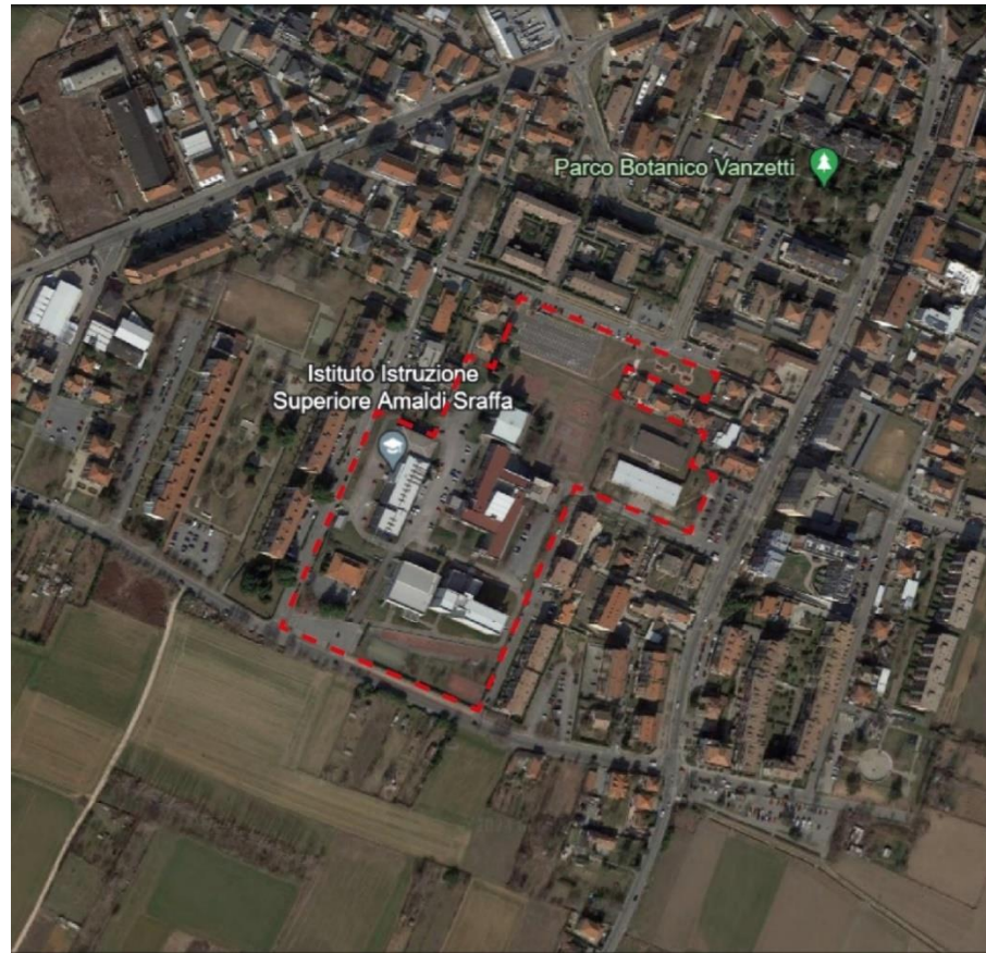
Figure 17 Top view of the site. Google (2024) Orbassano
