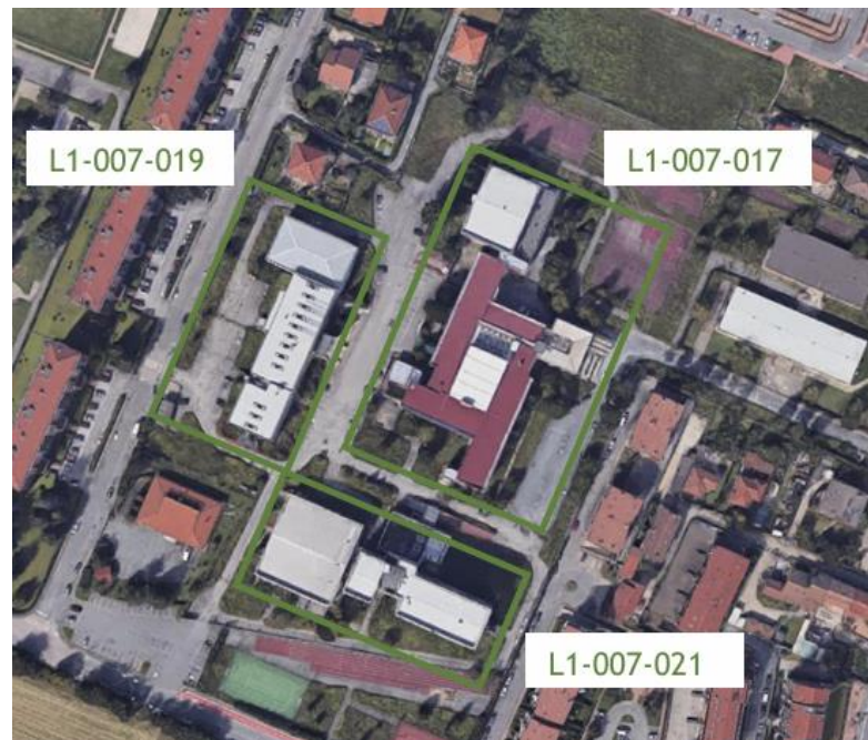
Figure 25 Area of the school complex under review with identification of the three buildings codes (source: Energy Diagnosis of 6-12- 2017, L1-007-017_019_021)
