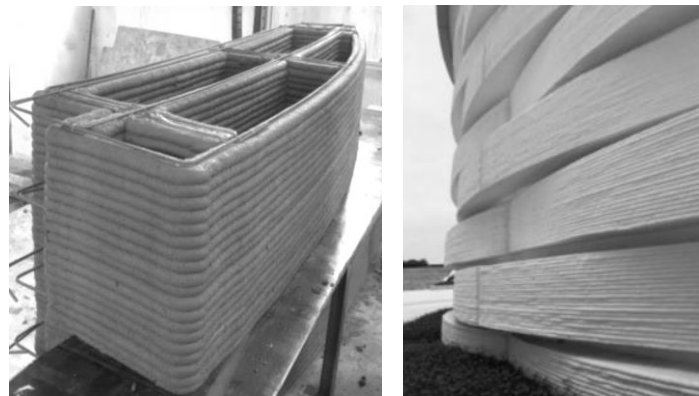
Image 1 3D printed elements: wall segments printed in factory and completed fabricated 3D printed concrete building in Nanjing. Source: (Khan, Sanchez, & Zhou, 2020).
