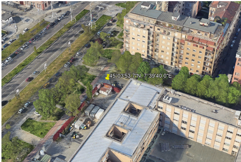
Figure 5.4: Static dataset location (yellow pin) on Google Earth, near Politecnico di Torino, Corso Castellidaro (45°03'53.7"N, 7°39'40.0"E)
