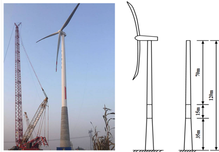
Figure 18: Wind Turbine Tower [71].
