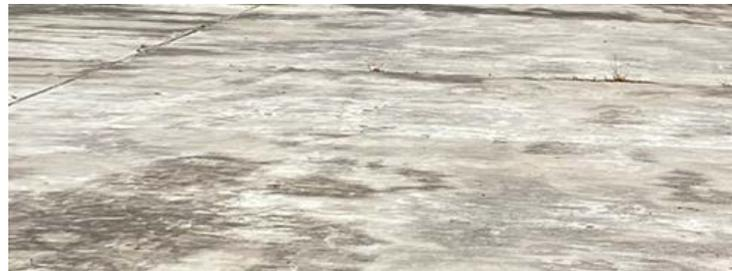
Figure 171 (Left) Efflorescence formation on the ceiling of the water tower. Photograph taken by Wassim Naghi, 2022. Retrieved from UNESCO Nomination Text, 2022, p. 62. (Right) Efflorescence formation on the reflective pools. Photographed by Nour Tabet, August 2024.
