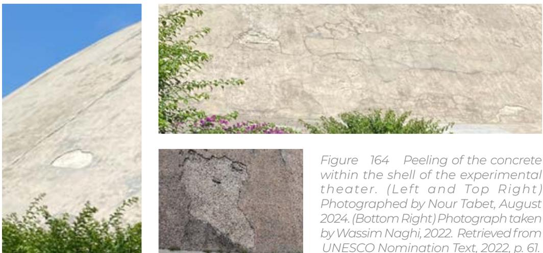
Figure 164 Peeling of the concrete within the shell of the experimental theater. (Left and Top Right) Photographed by Nour Tabet, August 2024. (Bottom Right) Photograph taken by Wassim Naghi, 2022. Retrieved from UNESCO Nomination Text, 2022, p. 61.
