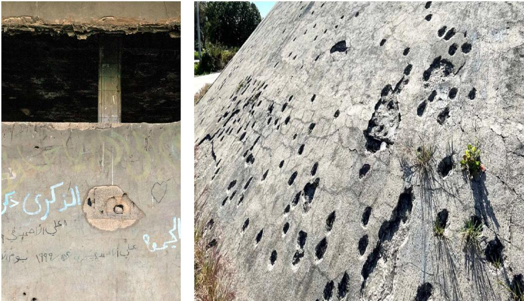
Figure 166 New openings created during the military presence on site in the administration building. Photographed by Ieva Saudargaitė, 2023. (Right) Bullet holes on the exterior shell of the Experimental theatre. Photographed by Maya Hmeidan, 2024. Retrieved from UNESCO Conservation Management Plan, 2024, p.191 & 142.
