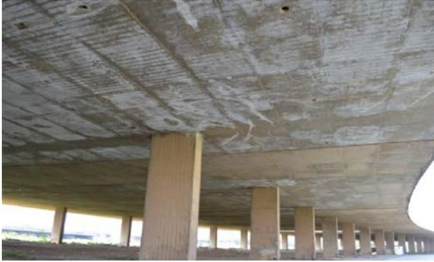
Figure 170 (Top) Efflorescence formation on the ceiling of the northern portion of the Great. Photographed by Sanaa Abdallah 2015. Retrieved “LA FOIRE INTERNATIONALE DE TRIPOLI.”, 2015, p. 22. (Bottom Left) Efflorescence formation on the ceiling of the experimental theater. Photographed by Nour Tabet, August 2024. (Bottom Right) Black crust and efflorescence formations on the interior of the Manege. Photographed by Nour Tabet, August 2024.
