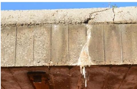
Figure 172 Calcareous deposits in the fractures within the ceiling of the ticket booth. Photographed by Sanaa Abdallah 2015. Retrieved “LA FOIRE INTERNATIONALE DE TRIPOLI.”, 2015, p. 15.
