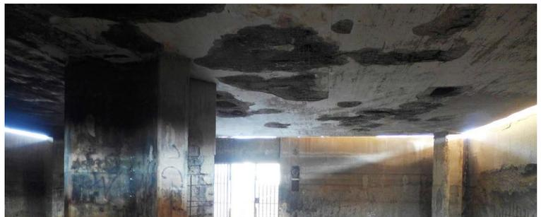
Figure 159 Severe blistering within the ceiling of the basement floor of the Helipad. (Left) Photographed by Pamela Jerome, 2019. (Right) 2022. Photographed by Maya Hmeidani, 2018. Retrieved from UNESCO Conservation Management Plan, 2024, p. 167.
