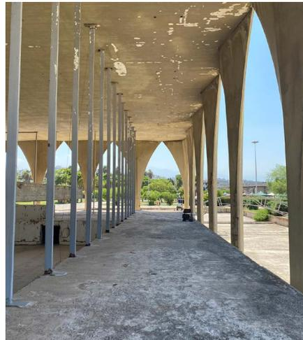
This building was nearly completed in 1975. Unfortunately, due to looting and lack of maintenance, all finishing elements were lost. The pavement, glazing, doors, and fixtures are no longer present just as the steel frames are corroding.
