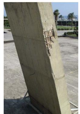
Figure 160 (Left) Blistering in several spots within the Arch of the Amphitheater. Photographed by Nour Tabet, August 2024. (Left) Peeling, blistering, and thin or missing areas of coating. (Right) Spalled concrete near a construction joint. We can see the effect of blistering here as well. Retrieved from RKIF Grand Arch and Open-Air Theatre Final Report, May 22, 2023, WJE No. 2022.4235.1, p. 15-17.
