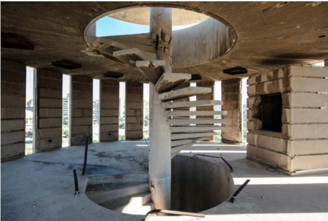
Figure 129 The interior of the water tower's third level, showing the staircase leading to the panoramic platform. The central column supporting the Water Tower's roof is deteriorated. Photographed by Ieva Saudargaite, 2023. Source: UNESCO Conservation Management Plan, 2024.
