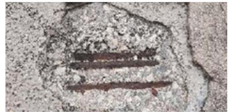
Figure 158 Blistering within the exterior of the dome of the experimental theater. Photograph taken by Wassim Naghi, 2022. Retrieved from UNESCO Nomination Text, 2022, p. 61.
