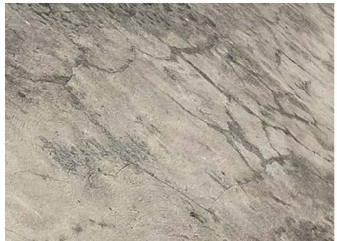
Figure 152 Network of thin cracks within the dome of the experimental theater. Photographed by Nour Tabet, August 2024.
