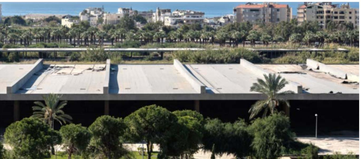
Figure 113 From the top, one can see the Boomerang's waterproofing membrane that is in a deteriorated state and needs replacement. Photographed by Ieva Saudargaite, 2023. Source: UNESCO Conservation Management Plan, 2024.
