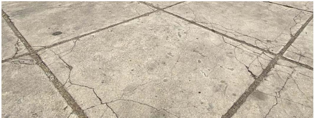
Figure 151 Fractures within the main entrance pavement. Photographed by Nour Tabet, August 2024.
