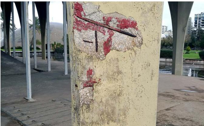
Figure 162 (Left) Fragments have already fallen and exposed the steel. Lebanese Pavilion. Photographed by Mazen Haidar, 2019. Retrieved from UNESCO Conservation Management Plan, 2024, p.160. (Bottom) Cracking of the external thin layer of mortar covering the reinforced concrete. Photographed by Maya Hmeidan, 2024. Retrieved from UNESCO Conservation Management Plan, 2024, p. 164.
