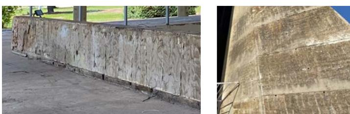
Figure 165 ( L e f t ) Differential erosion of the marble balustrade in the Lebanese pavilion. (Right) Differential erosion of the concrete shell of the Manège. Photographed by Nour Tabet, August 2024.
