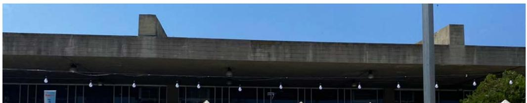
Figure 175 Soiling on the edge of the roof of the great canopy. Photographed by Nour Tabet, August 2024.
