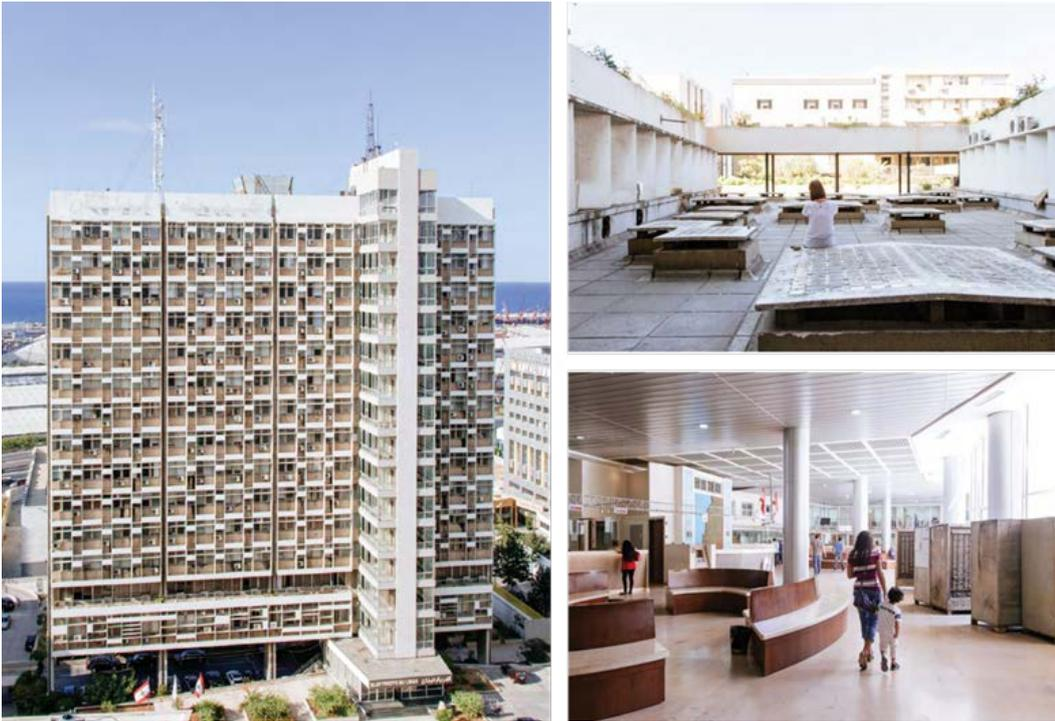
Figure 08 *Electricité du Liban (EDL)*. In 1966, a competition was created for the design for the EDL headquarters. The winning design was a proposal by Pierre Neema that featured a raised form held by pre-stressed concrete columns, creating a free-flowing floor plan and a clear unobstructed view of the Mediterranean Sea. Photographed by Dalia Khamissy, 2017.
