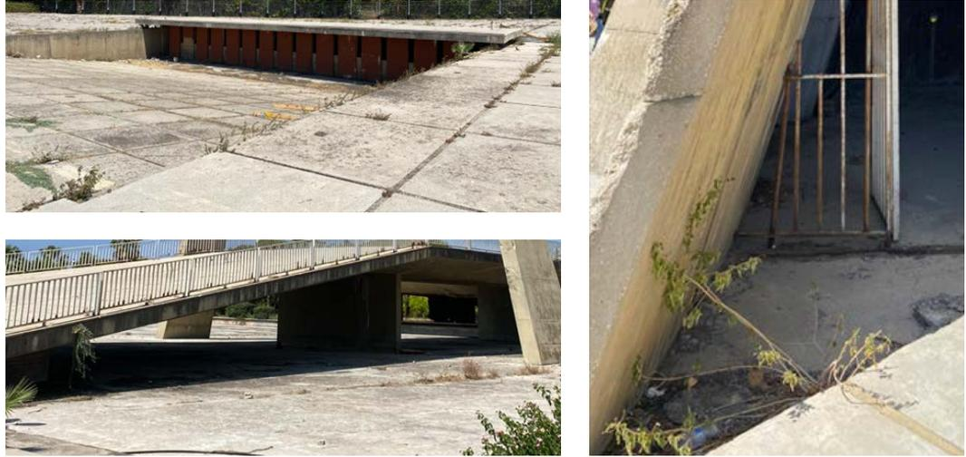
Figure 179 (Top Left) Plant growth between the tiles near the ticket booth. (Bottom Left) Plant growth within the concrete near the amphitheater. (Right) Plant growth within the concrete floor of the Manege. All photographed by Nour Tabet, August 2024.
