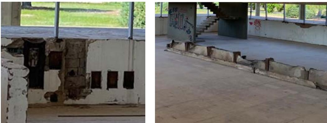
Figure 167 (Left) Missing portion of a wall in the Lebanese pavilion. (Right) Missing partition wall within the lower floor of the Lebanese pavilion. All photographed by Nour Tabet August 2024.
