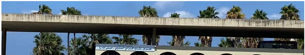
Figure 174 Soiling on the edge of the roof of the entrance portico. Photographed by Nour Tabet, August 2024.
