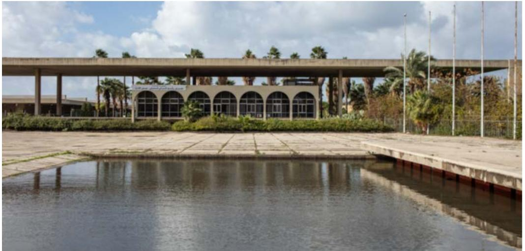
Figure 96 The ticket booth floods with water after heavy rainfall due to the lack of maintenance. Photographed by Ieva Saudargaite, 2023. Source: UNESCO Conservation Management Plan, 2024.
