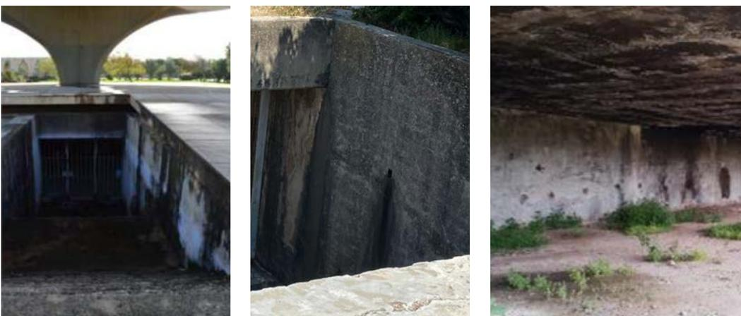
Figure 178 (Left) Mold growth on the walls of the helipad's underground. Photographed by Sanaa Abdallah 2015. Retrieved “LA FOIRE INTERNATIONALE DE TRIPOLI.”, 2015, p. 33. (Center) Mold growth on the walls of the basement of the experimental theater. Photographed by Nour Tabet, August 2024. (Right) Mold growth on the ceiling and walls of the customs department. Photograph taken by Wassim Naghi, 2022. Retrieved from UNESCO Nomination Text, 2022, p. 63.
