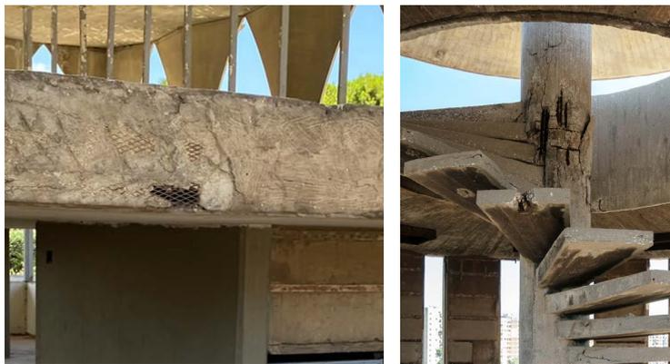
Figure 163 ( L e f t ) Peeling of the concrete in the slab in the Lebanese Pavilion. Photographed by Nour Tabet, 2024. (Right) Peeling of the concrete within the central column of the water tower. Photographed by Ieva Saudargaite, 2023. Retrieved from UNESCO Conservation Management Plan, 2024, p.177.
