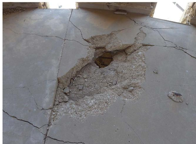
Figure 156 Evidence of the Civil War throughout the site needs to be carefully evaluated and potentially preserved and interpreted. In the Water Tower, there is damage to the slab from an unexploded ordnance. Photographed by Pamela Jerome, 2019. Retrieved from UNESCO Conservation Management Plan, 2024, p.230
