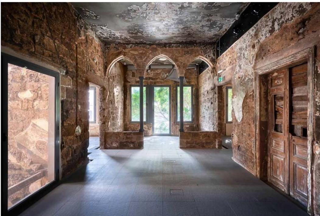
Figure 183 Figure 2. Inside Beit Beirut. Original damage by war and time is preserved. Instead of fixing structural damage in a way to restore things as they had been, new structural interventions were made distinct while damages were kept intact. Photographed by Roman Robroek, April 12, 2022. Retrieved from <https://romanrobroek.nl/i-photographed-the-beit-beirut-building-in-lebanon/>.
