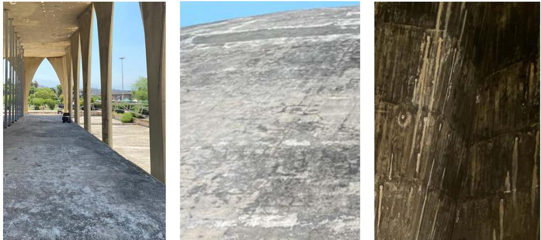
Figure 169 (Left) Crust formation on the floor of the Lebanese pavilion. (Center) Crust formation on the shell of the experimental theater. (Right) Black crust and efflorescence formations on the interior of the Manege. All photographed by Nour Tabet, August 2024.
