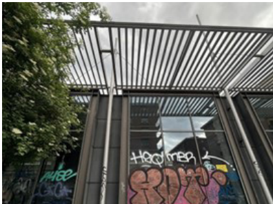
Figure 24 Steel and glass façade, photographed by the author
