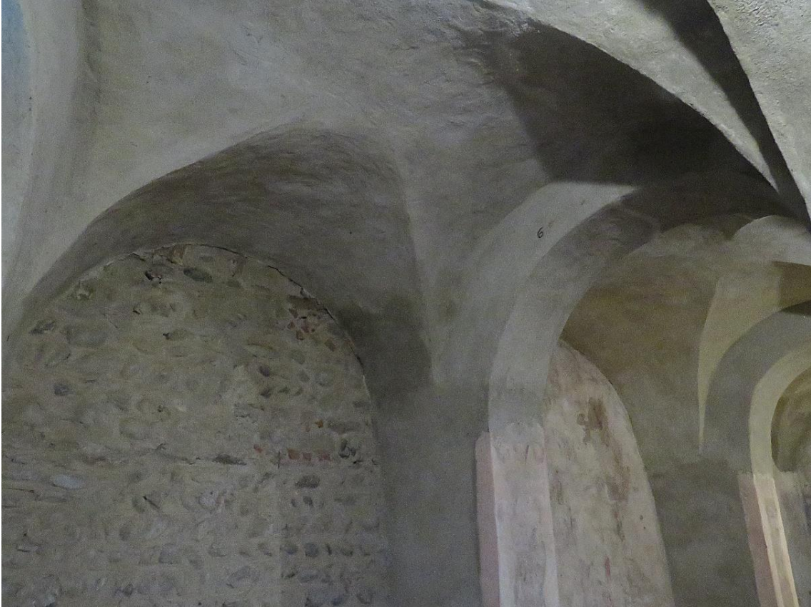
Image 7 - Groin vault in the side nave of the Santo Stefano church: Masonry structure with plaster finishes.
