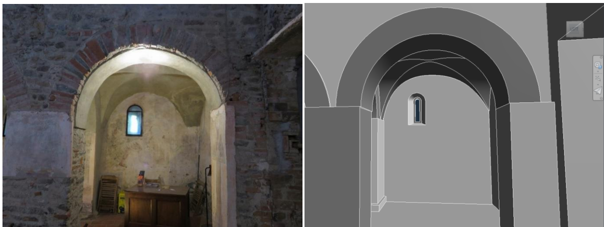
Image 46 - Arch on the nave wall in the church (left) and its virtual representation on the model done with in-situ tool (right).
