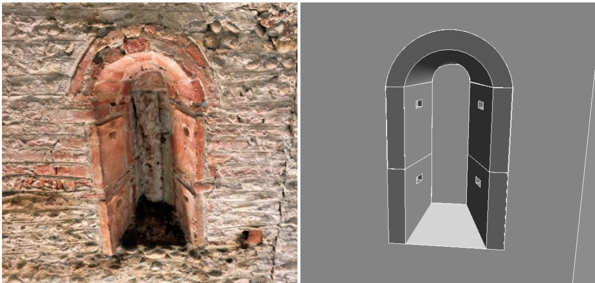
Image 50 - Niche on the entrance wall in the church (left) and its virtual representation on the model done with in-situ tool (right).
