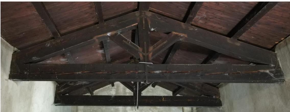
Image 8 - Wooden trusses supporting the central nave roof of Santo Stefano Church.
