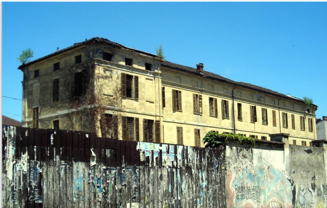
Figure 9. Buon Pastore Institute before renovation (view from Via Moris)
