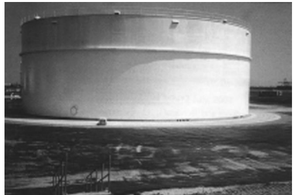
Figure 1-4: Example of unanchored storage tank (Courtesy of D&H Group)
