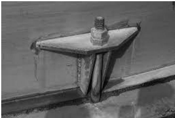
Figure 1-3: Example of anchor (Courtesy Vathi & Karamanos)
