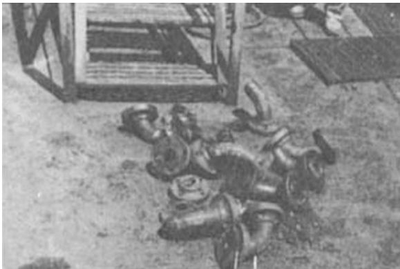
Figure 1-10: Damage to piping connections [4]
