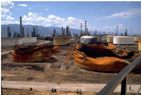
Figure 1-5: Tank farm with some tanks destroyed by fire in Tüpras refinery [6]
