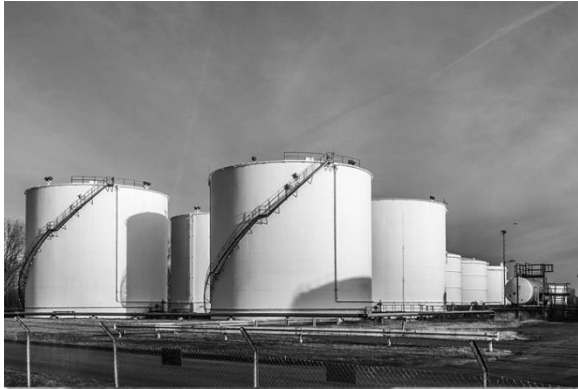
Figure 1-1: Example of above-ground storage tank (Courtesy of SIS GmbH)
