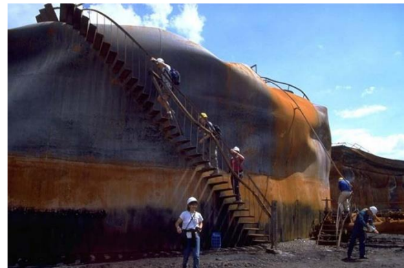
Figure 1-6: Thermal buckling due to heat radiation [6]
