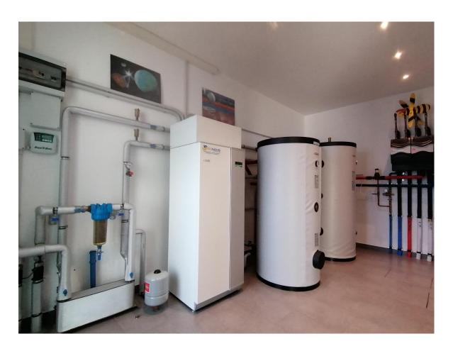
Figure 35 Heat pump NIBE F12345 and buffer tank
