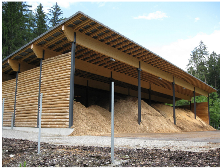
Figure 2.3: Picture of an Open-air drying plant featuring a roof and covered on three sides[6]
