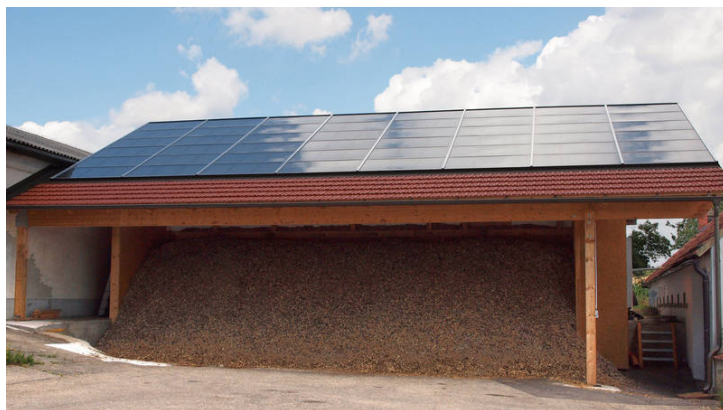
Figure 2.5: Picture of a solar based open air drying plant (equipped with solar-air collectors) [9]
