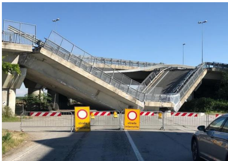
Figure 1-1 _ Collapse of Fossano bridge, 2017 (Micozzi et al., 2023)
