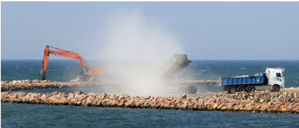
Figure 3 Breakwater under construction ( Leffmann )
