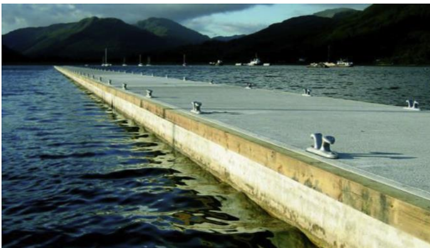
Figure 7 Box-type breakwater ( Jian Dai, 2018 )
