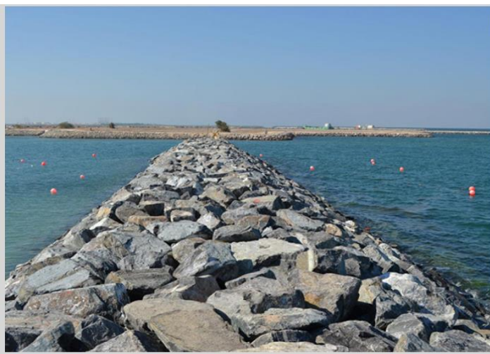
Figure 15 Rubble Mound Breakwater ( Breakwater Construction, n.d. )
