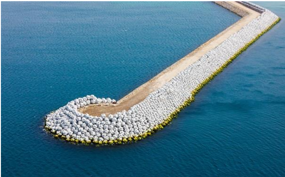
Figure 4 Remains of ancient breakwaters ( Rubble mound breakwater design example, 2024 )
