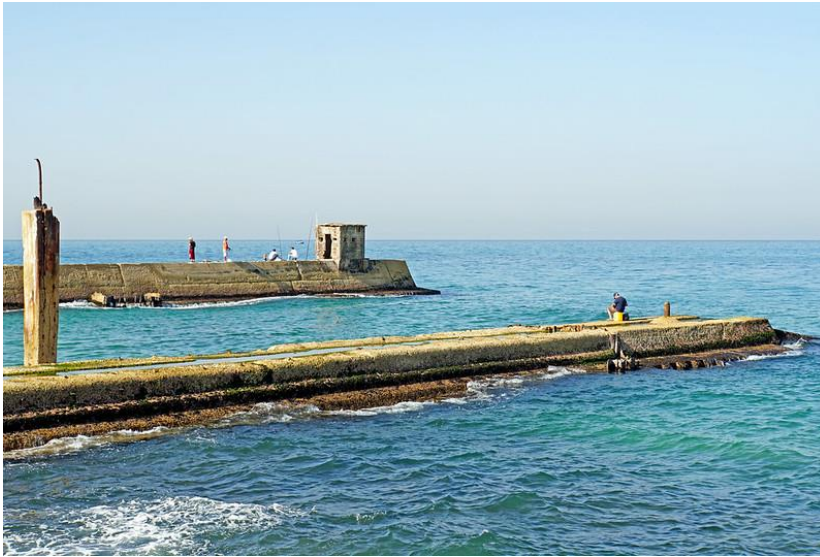
Figure 2 Old Port Breakwater ( Jarvis, Israel-04557 - Old Port Breakwater, 2017 )
