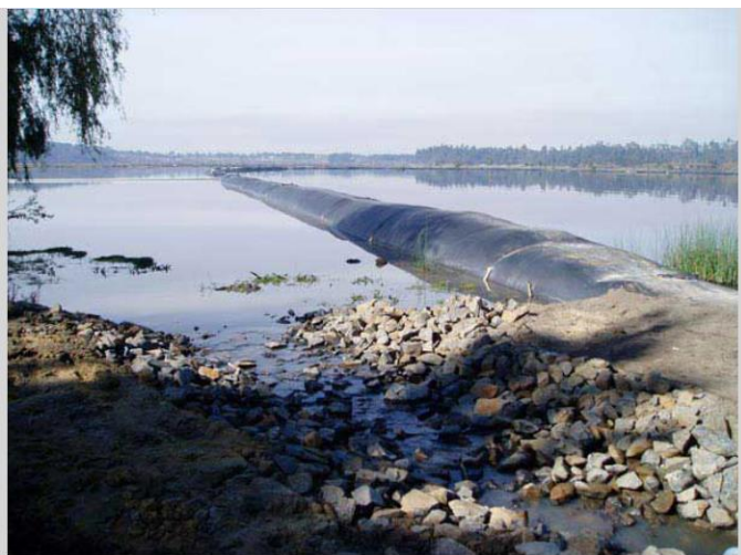
Figure 17 Geotextile Tubes ( Breakwater Construction, n.d. )
