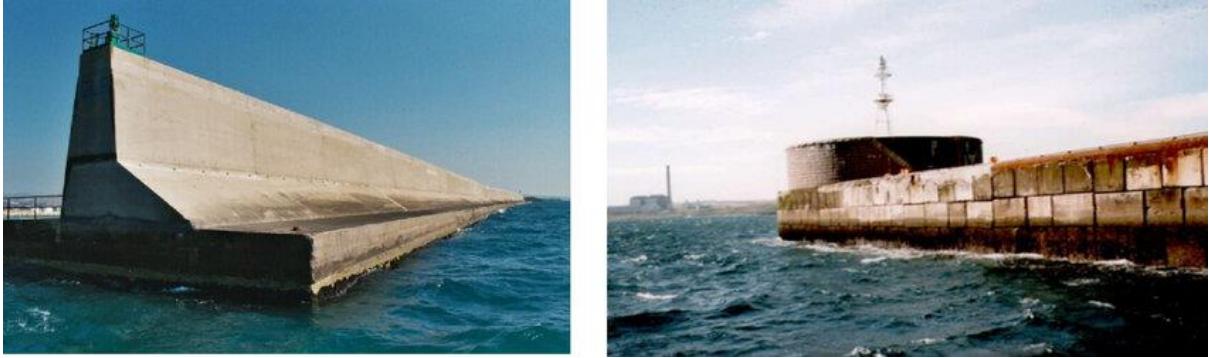
Figure 5 Example of Vertical Breakwater ( Bruce, 2017 )
