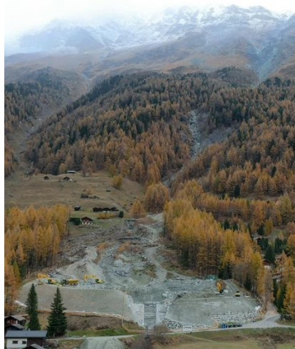
Figure 10 : Work at the retention basin on Pétérey torrent (2017)
