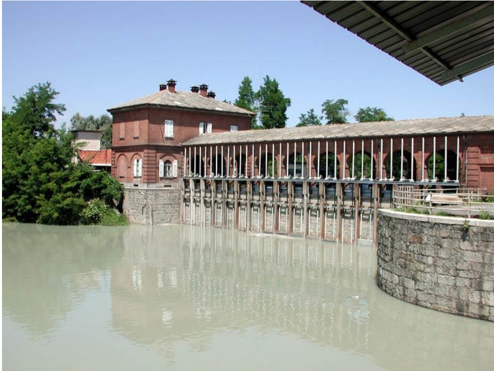
Figure 2.5, Canale Farini intake structure. Credit: Andrea Miola [15]
