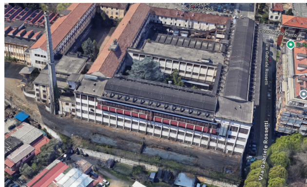
(b) Focus on the current state of the building subject of this analysis
