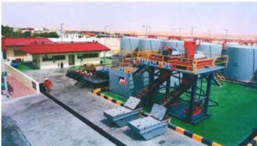
Figure 29: A View of Liquid Mud Plant
