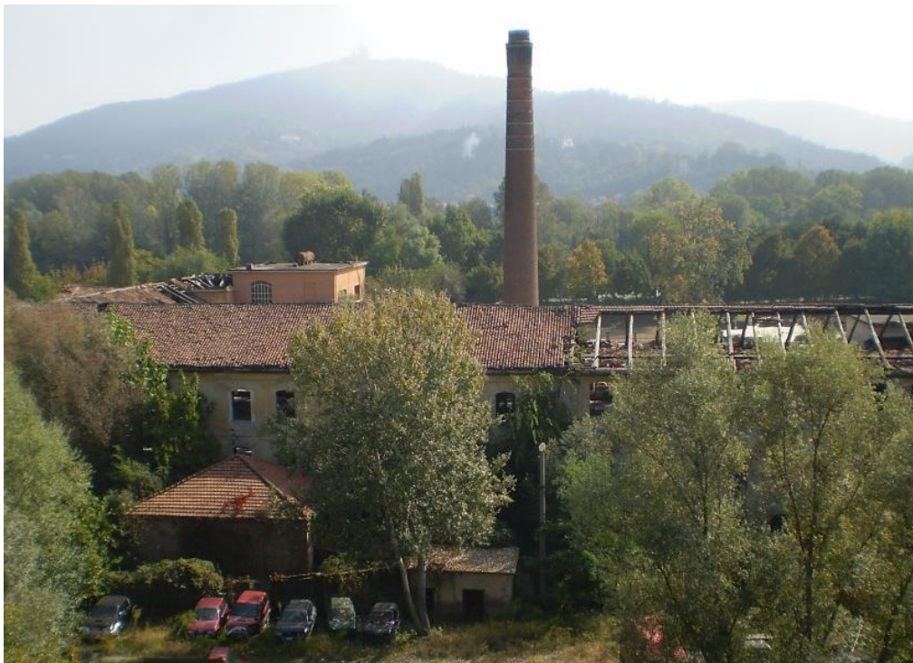
Figure 45 View of the Spinning Mill
