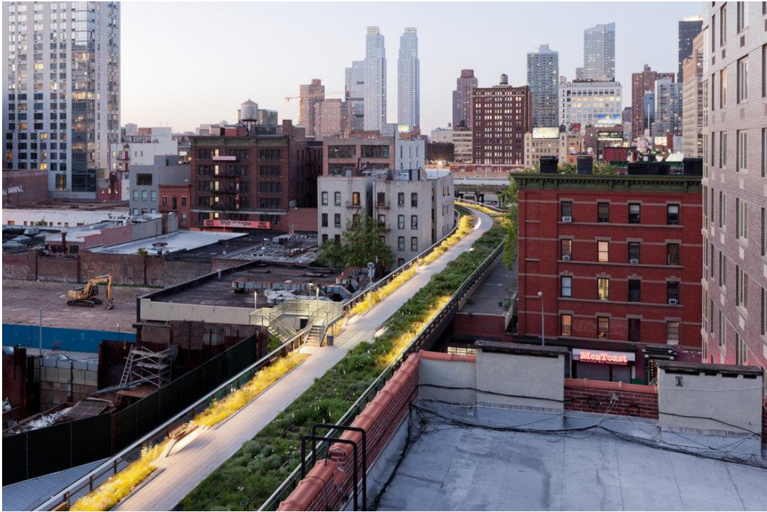
Figure 15 View of the High Line, passing through the Manhattan Skyline
