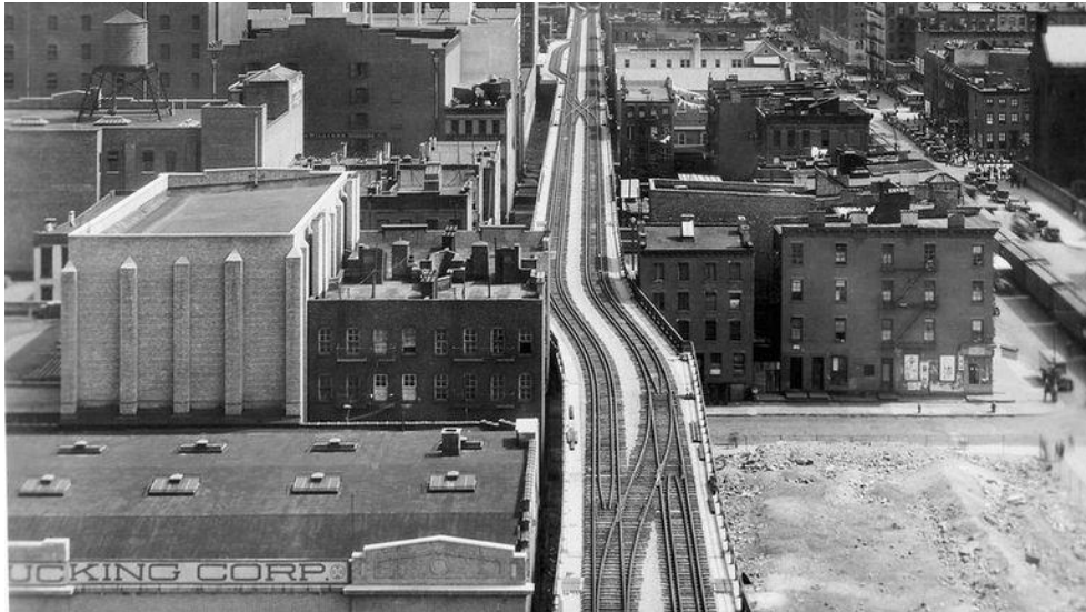
Figure 14 The Abandoned Rail-Line
