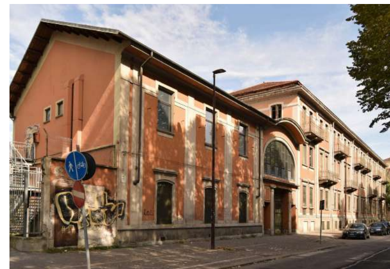
Fig. 45, Fig. 46_ Publicity campaigns. Source: https://www.design-is-fine.org/post/54826322680/walter-martiny-industria-gomma-sneakers-superga Fig. 47_ Current building. Source: https://fondoambiente.it/luoghi/ex-fabbrica-superga?ldc
