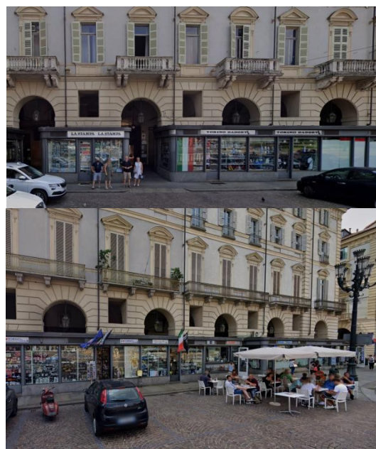
Figure 72 : Current shop situation at site 1
