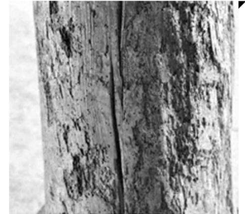
▲ **Fig. 44/** Column attacked by beetles. Source: Wang, s.: damage classification to historical wooden structures: a preliminary survey and recommendation for Dong minority drum towers, *int. Arch. Photogramm. Remote sens. Spatial inf. Sci.*, xlv-m-1-2021, 821–827, 2021 <https://doi.org/10.5194/isprs-archives-XLVI-M-1-2021-821-2021>
