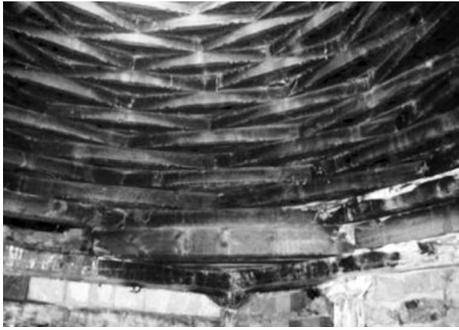
these dwellings from Lisitsian's survey<sup>13</sup> (Fig. 33), which mostly have parallel setting ceiling structure with unhewn logs supported by four freestanding wooden columns, rendering as primitive archetypes. Like Georgian houses, Karadam can be found with different ground placements, including the pit houses – analogues of Meskhetian dwellings, however, the level of wooden craftsmanship has not evolved here as much as in Northern territories. (Sumbadze, 92)
