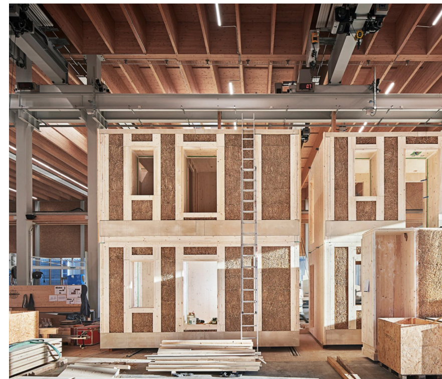
Fig 67 - Prefabricated elements for Bombasei, in Nänikon-CH, Source - Atelier Schmidt.
