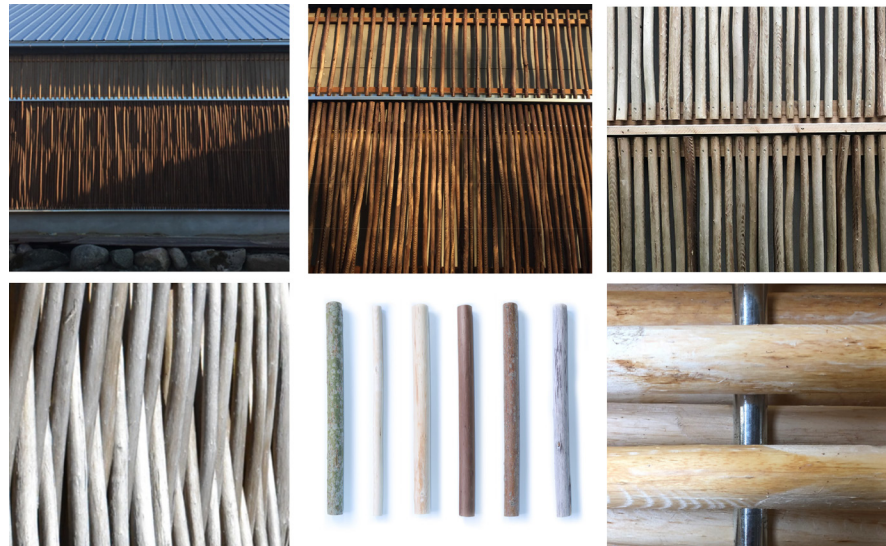
Fig 82 – Edited by author, façade systems made using uncut willow rods. Source – pilebyg.
