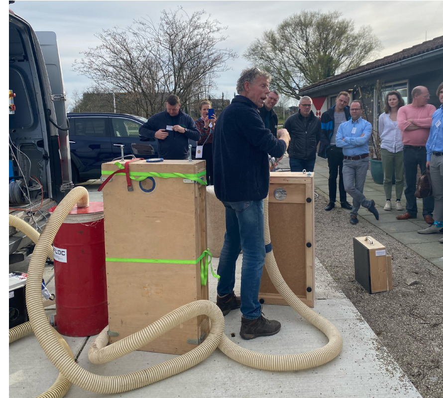
Blow-in straw instalation demo organised by Building Balance Organisation.
