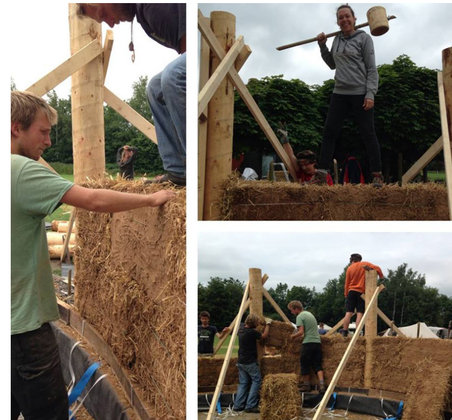
Fig 44 – Community-built Workshop Eco-house building with straw bales, Friesland. Source: mas con menos (making more with less).
