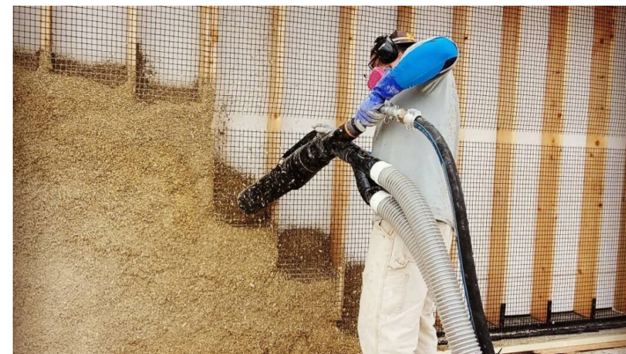
Fig 71 – Spray-applying cast-in-situ hempcrete, Source – HempBuild Magazine.
