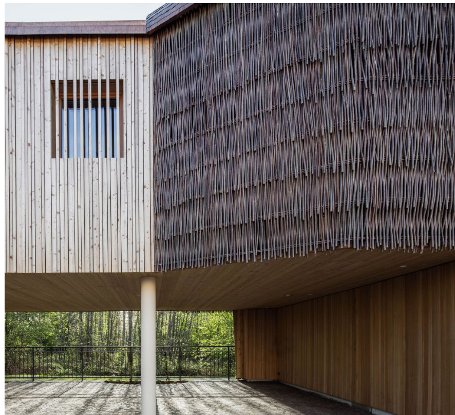
Fig 83 – RoSana Guest House, façade systems made using woven untreated and unpeeled willow wood. Source – Anna Heringer.
