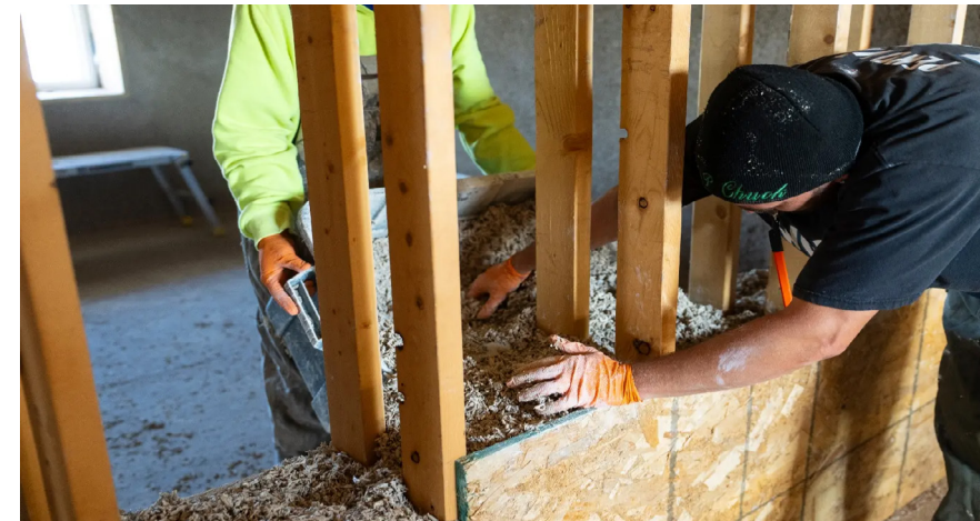
Fig 70 – Hand placing cast-in-situ hempcrete, Source – Grist. https://grist.org/indigenous/hempcrete-low-er-sioux-housing/
