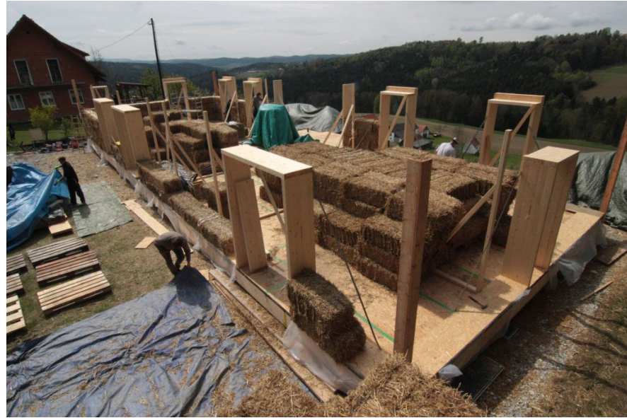
Fig 68 – The first load-bearing straw bale house in Austria with building permission, Source – European Straw Building Association.
