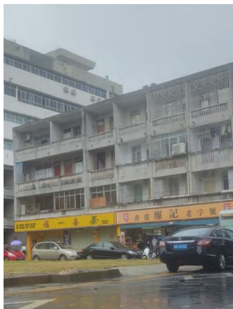
Figure 4-83 Photo of Street Wall d12 (Source: Photo by the Author)
