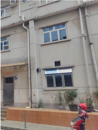
Figure 4-69 Photo of Street Wall c11 (Source: Photo by the Author)
