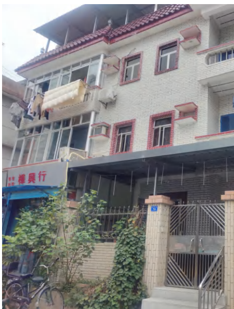
Figure 4-77 Photo of Street Wall c22 (Source: Photo by the Author)
