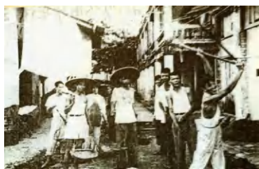
a) Repair the Road on China Side
