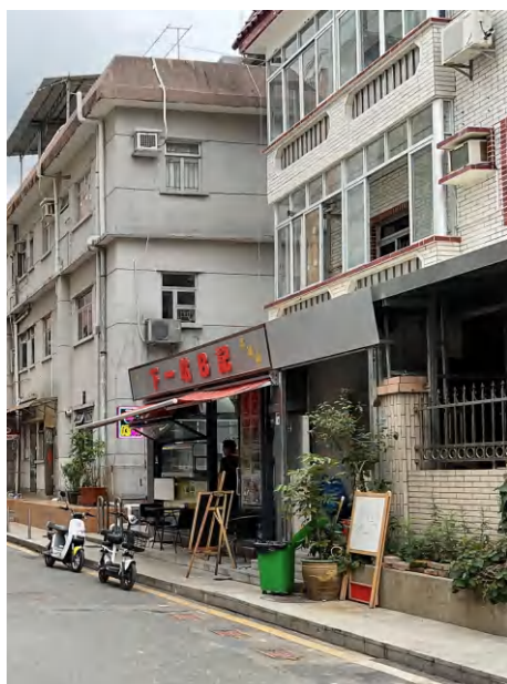
Figure 4-79 Photo of Street Wall c23 (Source: Photo by the Author)
