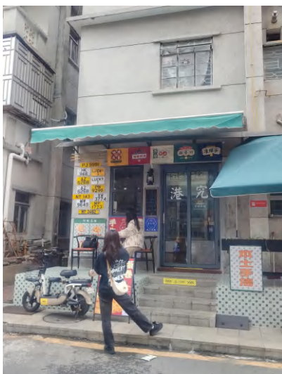
Figure 4-73 Photo of Street Wall c13 (Source: Photo by the Author)
