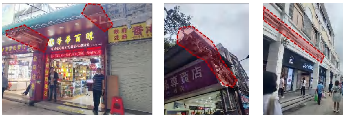
Hong Kong Drainpipe Hong Kong Monitor Shenzhen Wires
