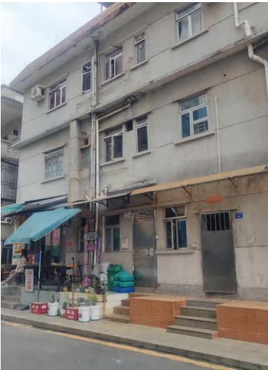
Figure 4-71 Photo of Street Wall c12 (Source: Photo by the Author)
