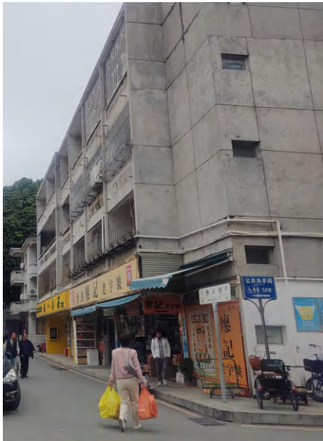
Figure 4-81 Photo of Street Wall d11 (Source: Photo by the Author)
