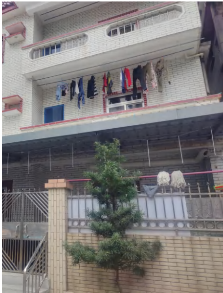
Figure 4-75 Photo of Street Wall c21 (Source: Photo by the Author)
