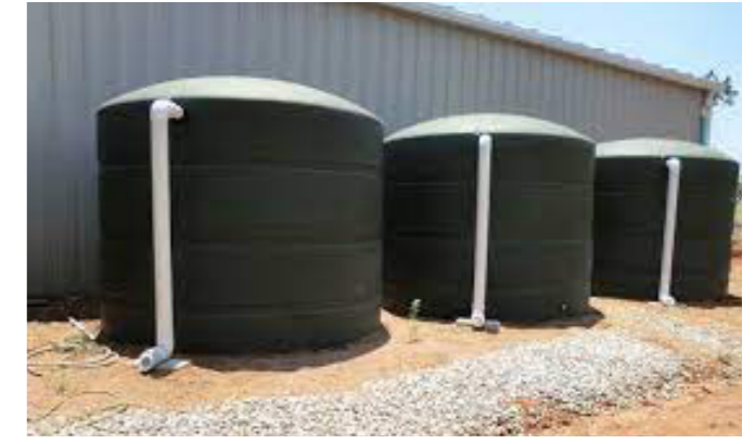
Figure 39 : Water storage tank
