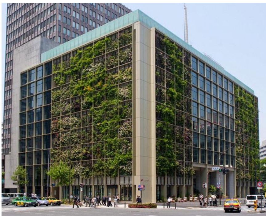
Figure 44: Pasona 02 planted green facade
