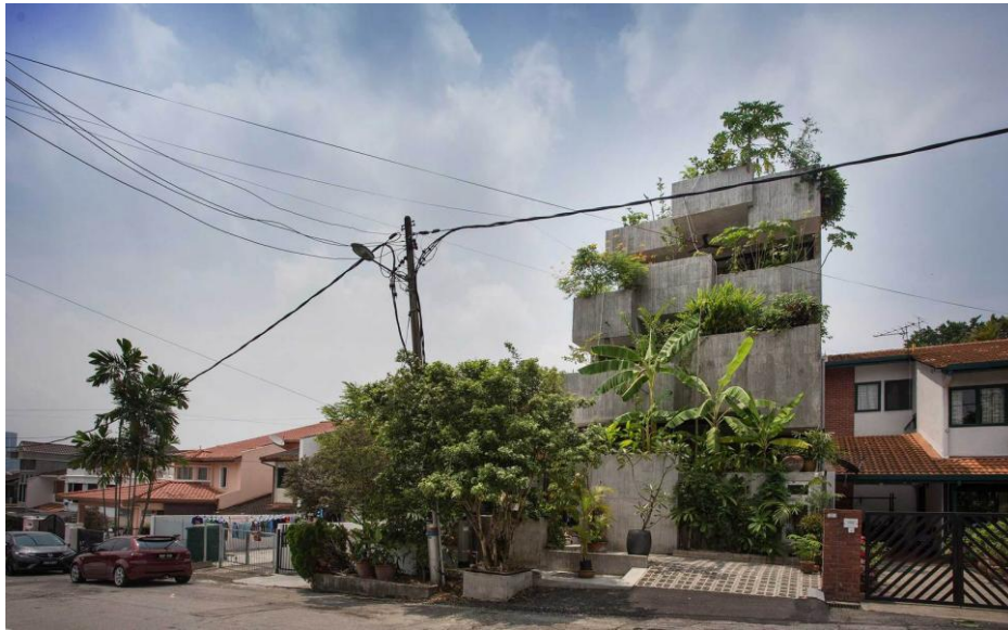
Figure 12: Planter Box House façade
