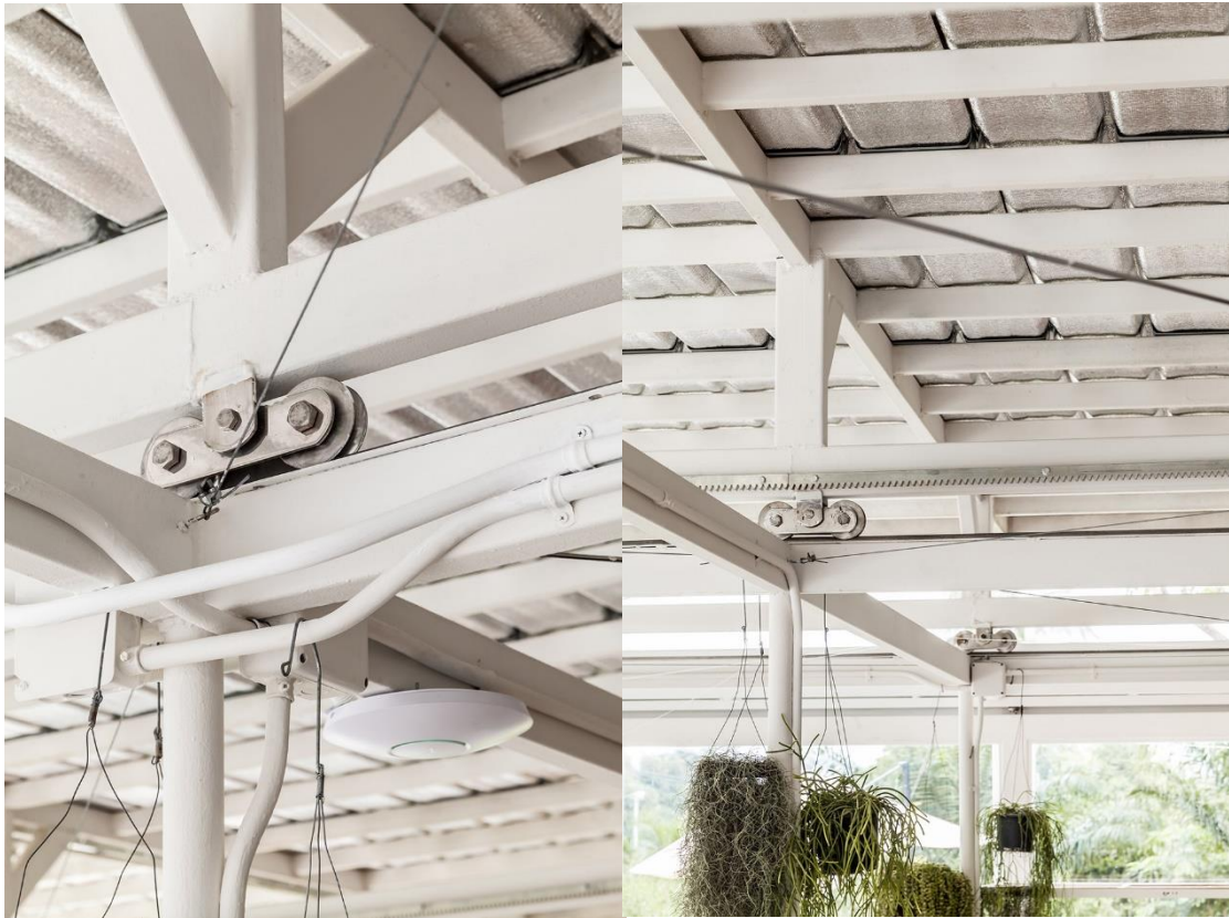
Figure 43: Sliding roof detail
