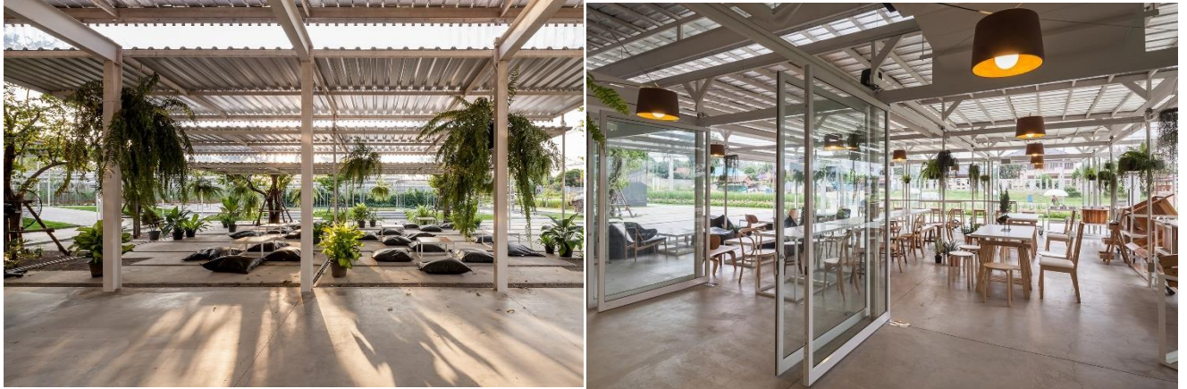
Figure 39: Moveable surfaces define different enclosures and the connecting open and enclosed spaces
