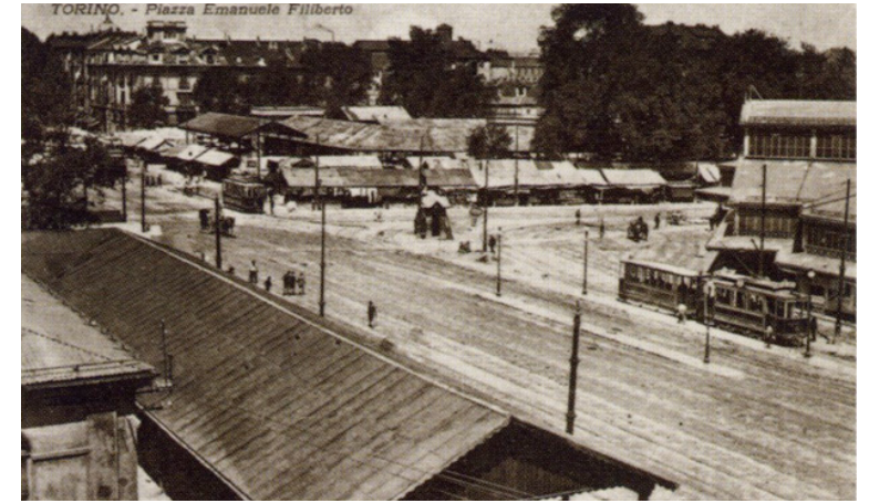
Fig.16 Vintage postcard. At the beginning of the twentieth century, the entire square was characterized by numerous canopies. in wood or metal carpentry, for the street vendors market source: (Coppo et al ., 2006)
