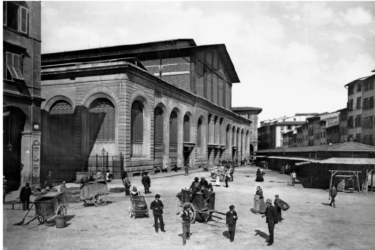
Fig.7 Mercato Centrale, Florence, 1870-1874, ca. 1890. Architect: Giuseppe Mengoni source: (Guàrdia & Oyón, 2015)
