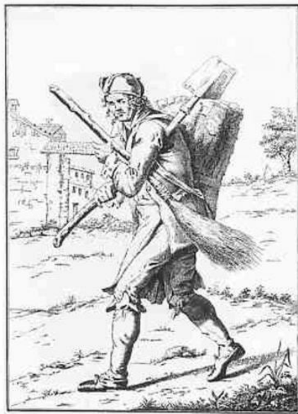
Figure 9: Waste and manure collector ( Ruee ). Source: (Lapini)
