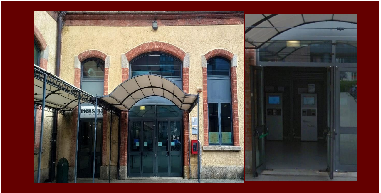
Figure 31: The entry kiosk of Canteen.
