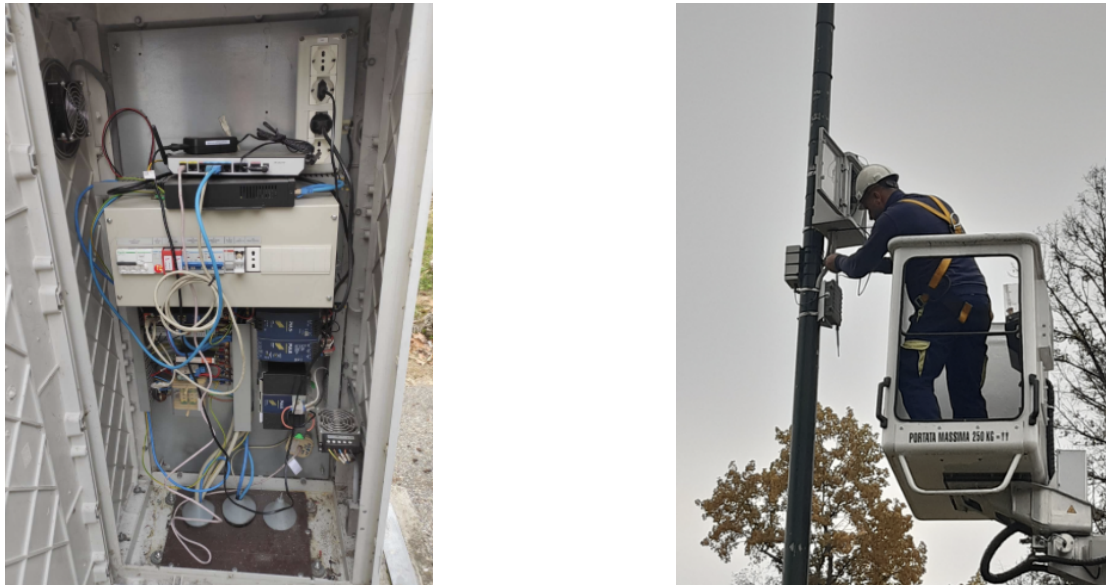
Figure 3.11: Installation of sensors in the target area
